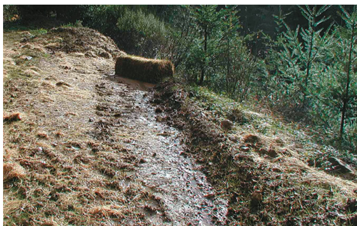
Straw bales or small heaps of slash can reduce stream sedimentation by slowing surface water and trapping sediment.
