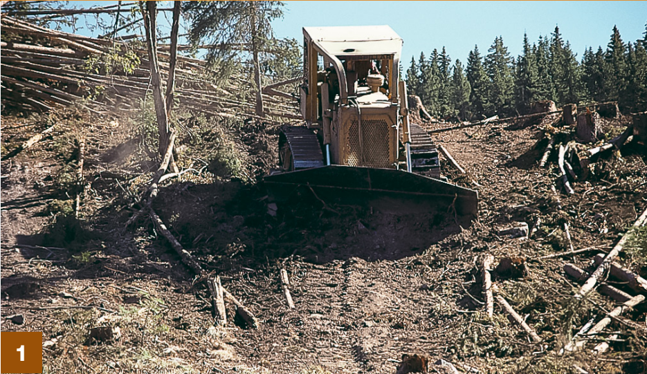
1 Begin construction of the skid trail cross ditch at the far edge of the skid trail.
