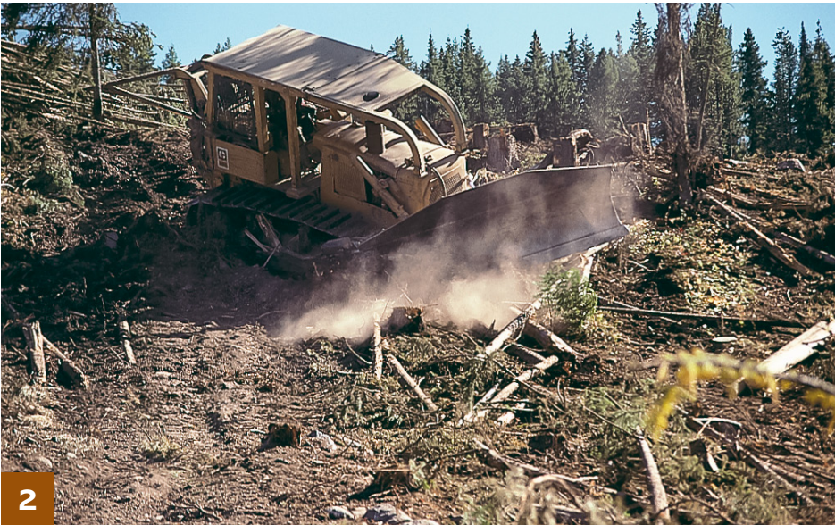
2 Cut an extra-deep cross ditch at an angle greater than perpendicular to the skid trail, and be sure the ditch is open so that water can drain out.
