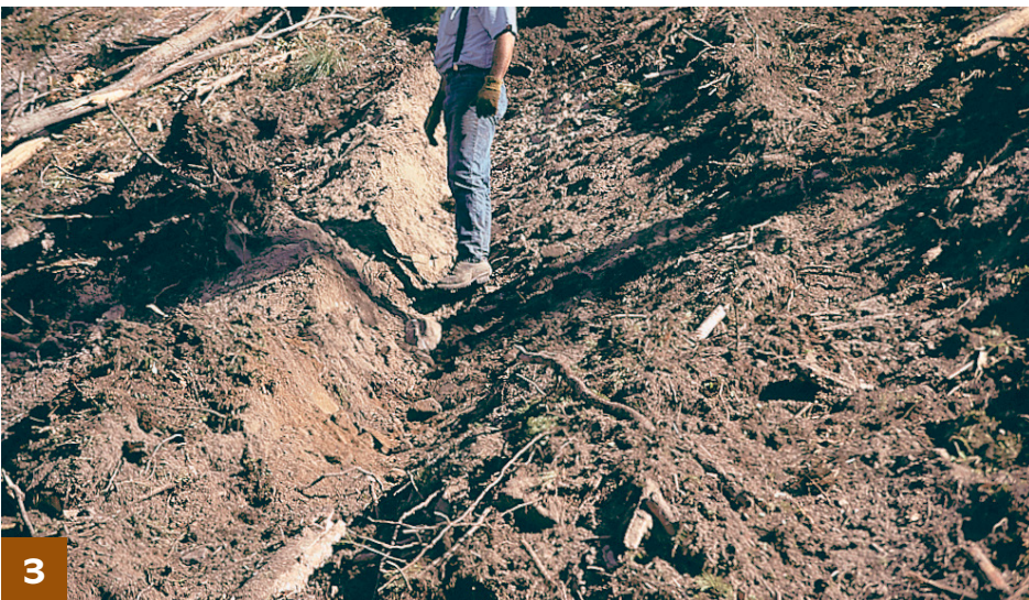
3 The finished skid trail cross ditch should be deep. This is more than a water bar.
