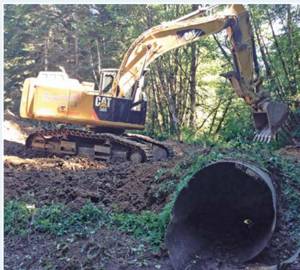
Removing the undersized culvert in Seeley Creek.
