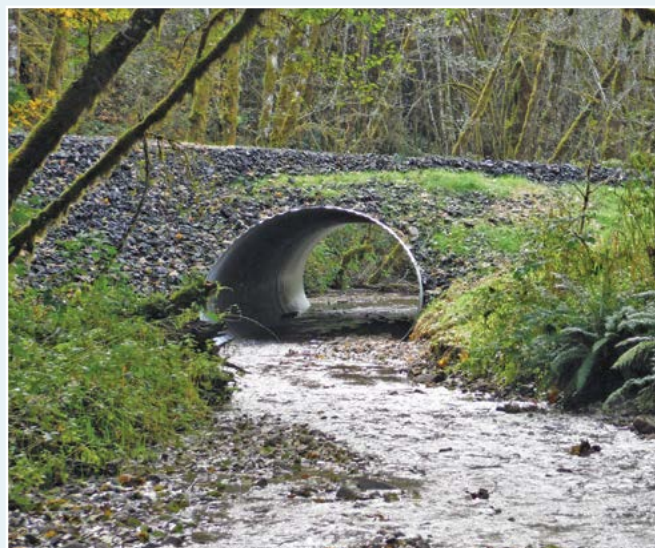
Finished culvert in Seeley Creek.
