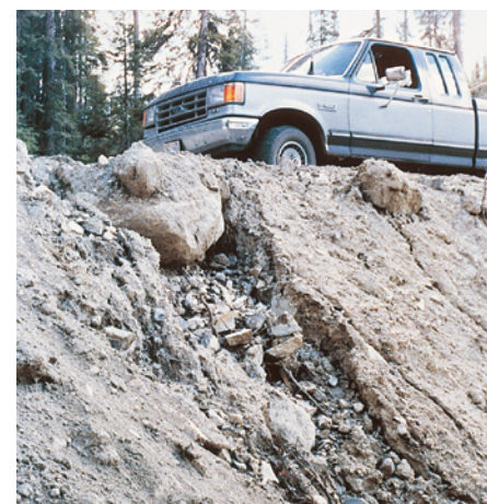
Soil sloughing off a road cut.
